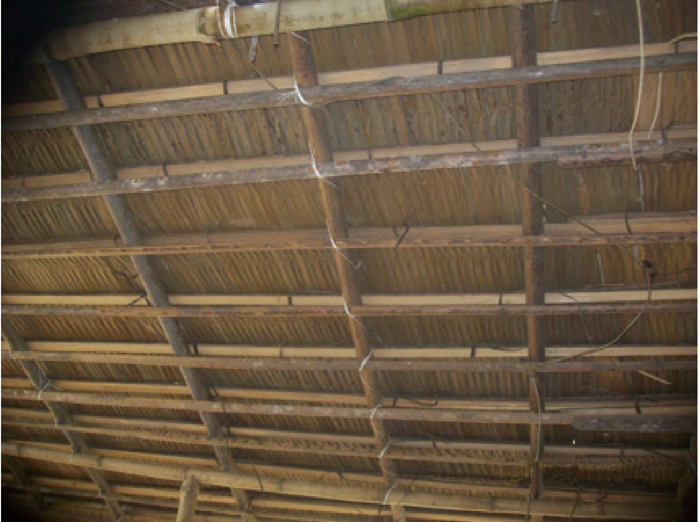
Figure 5: Inner part of a thatched roof.
