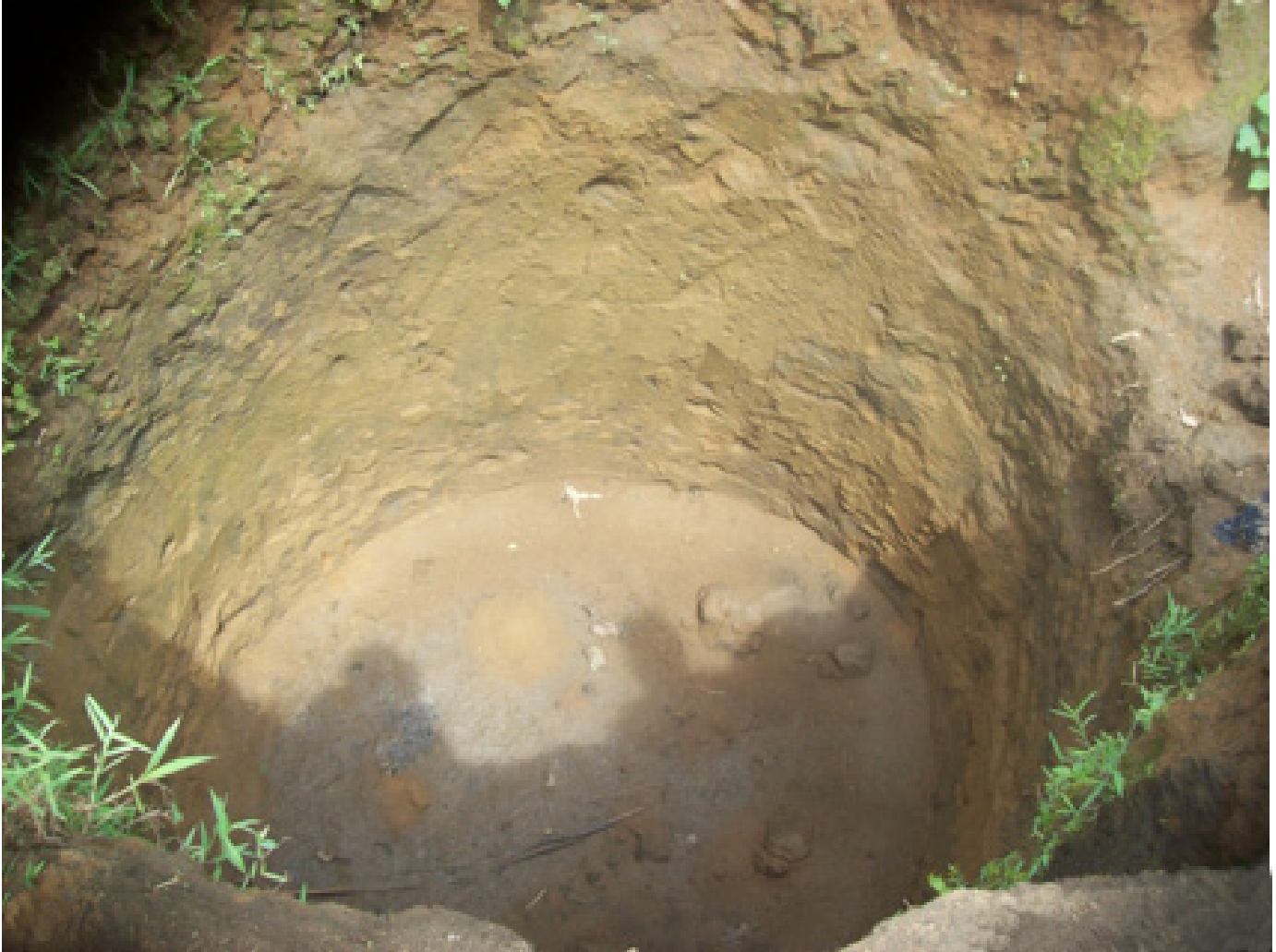
Figure 7: A pit for obtaining earth for construction.
